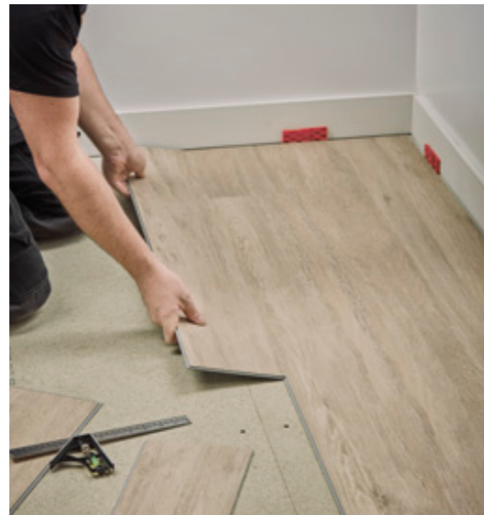
4. Continue to fit the rest of the floor, leaving a 5mm expansion gap. Skirting and colour matched scotias are available, see page 38 for more details.
