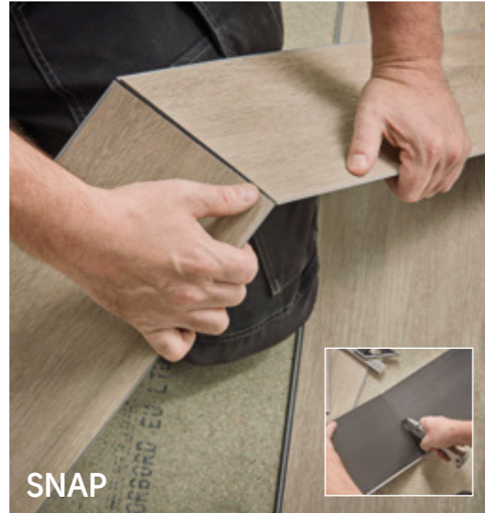
2. Snap the plank and use a utility knife to fully separate.
