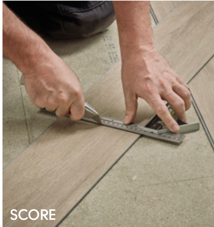
1. Using a knife and a straight edge, score the plank surface.
