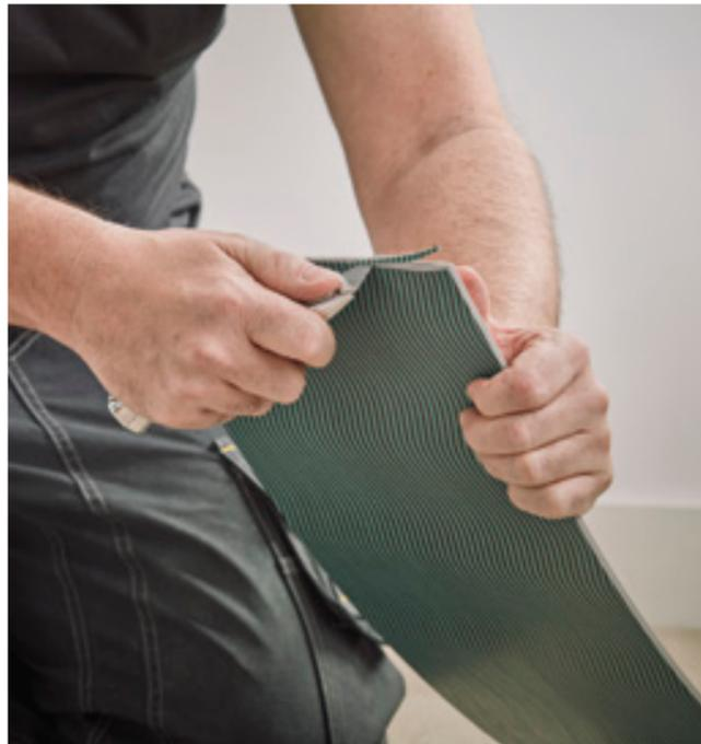
3. Using a knife, chamfer the cut edge to get a symmetrical sloping edge. The plank/tile will fit tight against the wall or another plank/tile.
