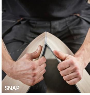
2. Snap the plank/tile surface. Use a knife to fully separate the plank/tile.
