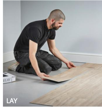
4. Lay the planks in place. The friction grip backing will hold the product to the floor. A tackifier around the edge of the room and at thresholds is recommended.\*\*
